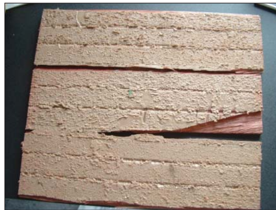
Figure 2 – Shear failure of MC adhesive from high timber movement.
