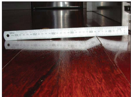
Figure 1 - Tenting in an overlay floor
