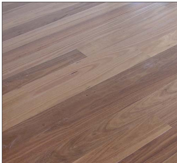
Engineered floor laid on acoustic underlay
